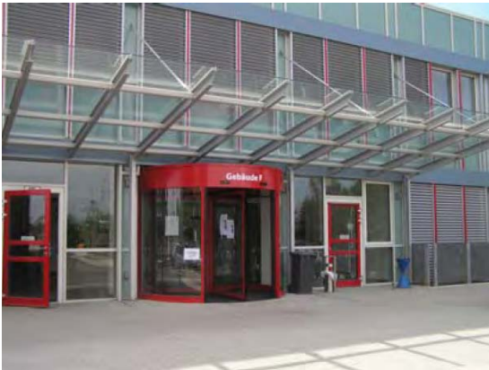
Main Entrance to Building F
